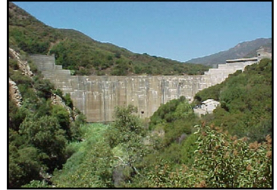
Matilija Dam in Ventura County, California
