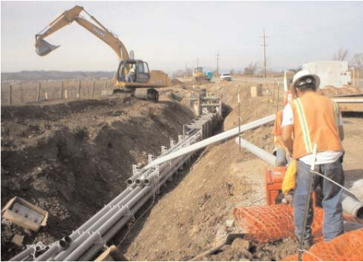
Tri-Valley Project: Conduit and tie-ins to vaults
