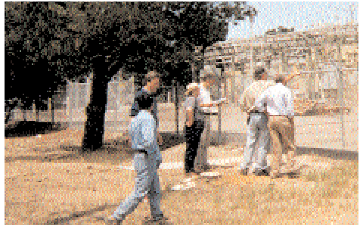
Aspen staff conferring at Tri-Valley 2002 Capacity Increase project
