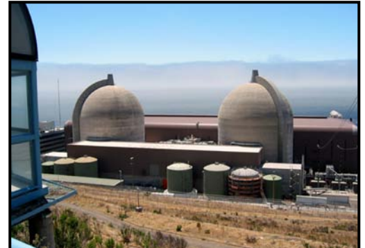
Diablo Canyon power plant is seeking to replace its steam generators.
