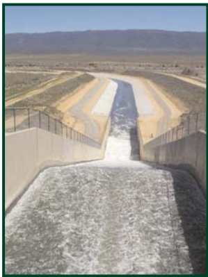
Cottonwood Chute - California Aqueduct East Branch
